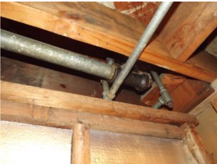
galvanized steel pipe
