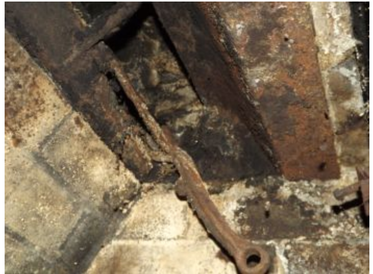
corroding damper
