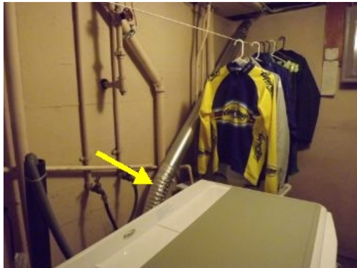
corrugated foil exhaust pipe
