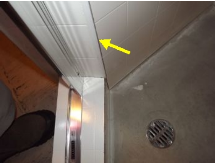
exposed edge of shower wall material
