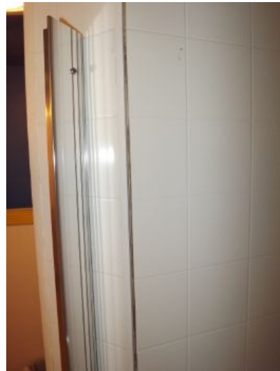
exposed edge of shower wall material
