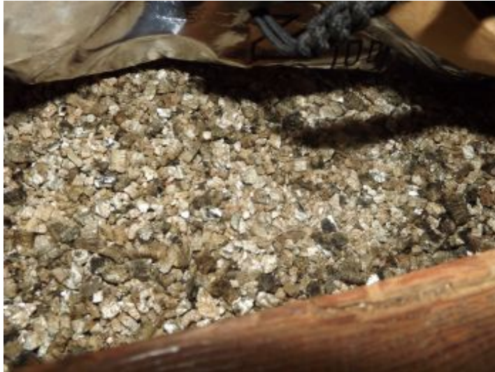
vermiculite insulation
