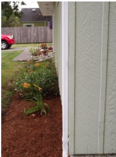
plants in contact with siding
