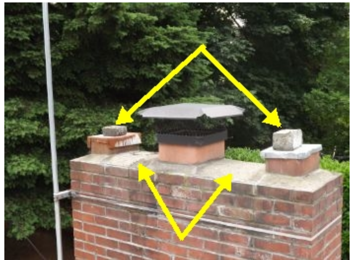
no chimney cap and unattached dead weights
