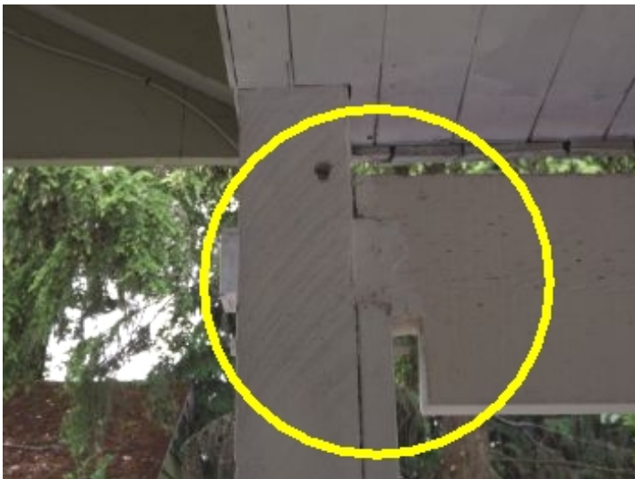
improvised beam attachment
