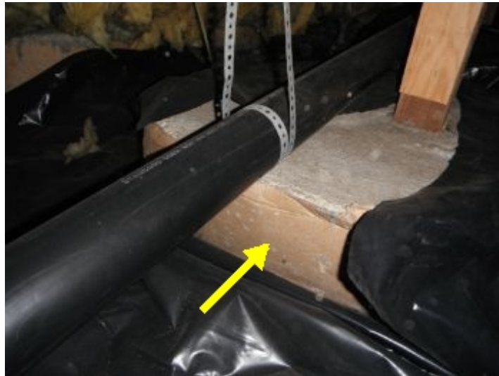
carboard form still in place
