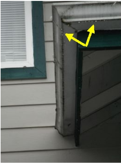
leaking gutter
