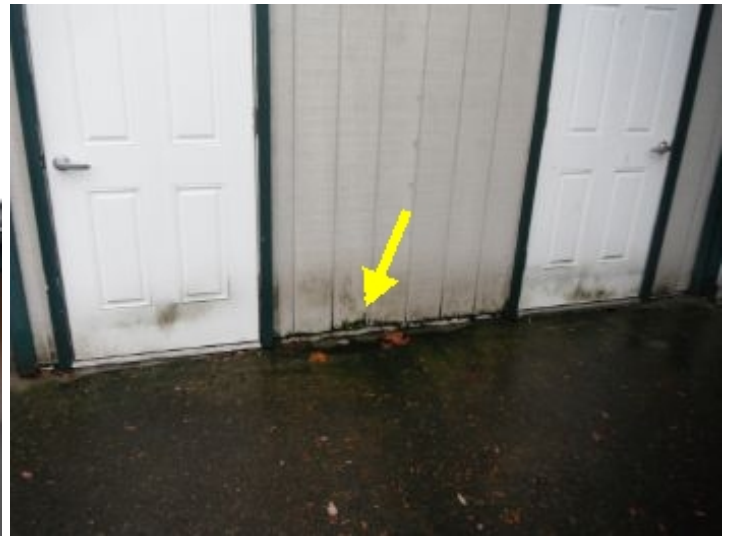
deteriorated siding
