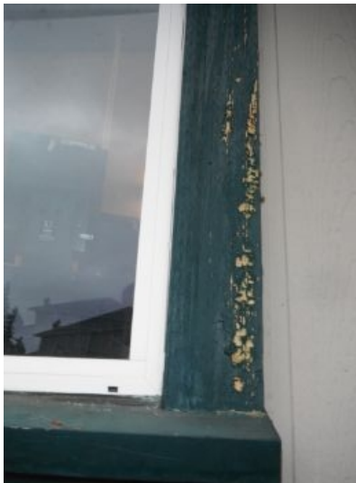
paint failing
