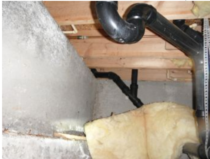
displaced insulation
