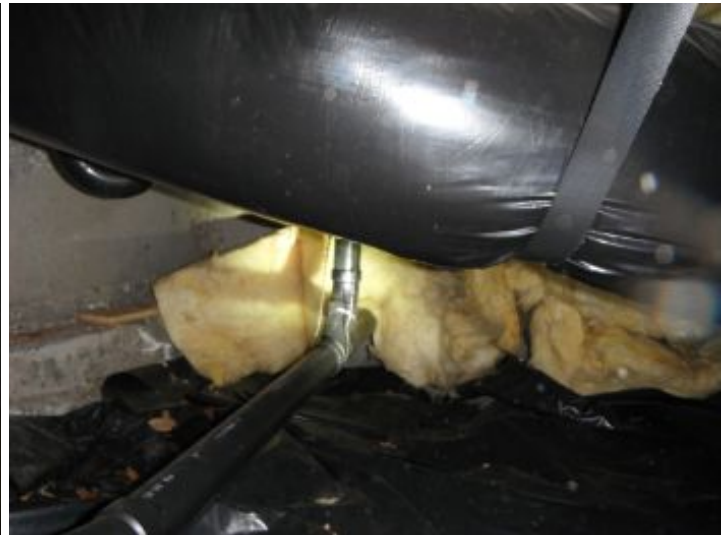
displaced insulation
